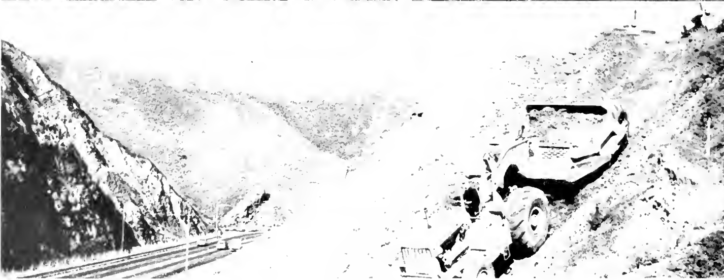
These photos courtesy of Caterpillar Tractor Company show construction on Walden Grade approach to Golden Gate Bridge. An ingenious and carefully worked out sequence of construction operations is being followed with the result that the work is being accomplished with minimum interference to passing traffic.
